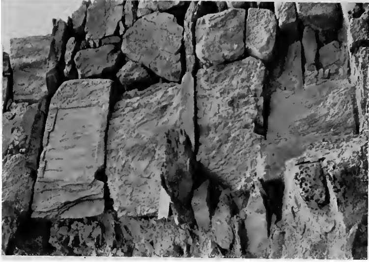
By the Author STONE FOR INSCRIPTION ON PIER OF SLUICE-GATES.
